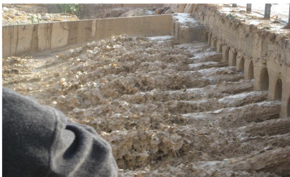
Fig. 2 Surface runoff in rainy day in Jericho (2008)
