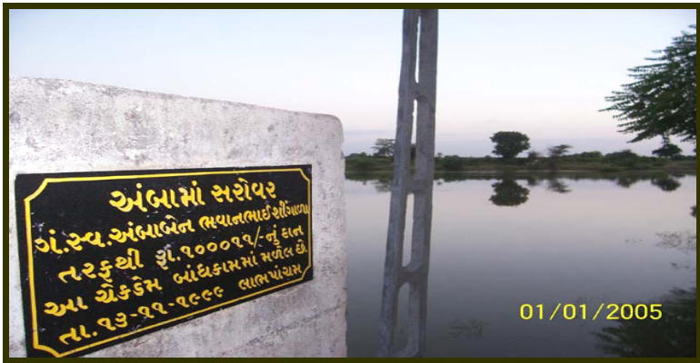
Fig. 6 Amba Sarowar, first check dam build near the village after Ambaben donated Rs. 1, 00,011/- for construction activity.
